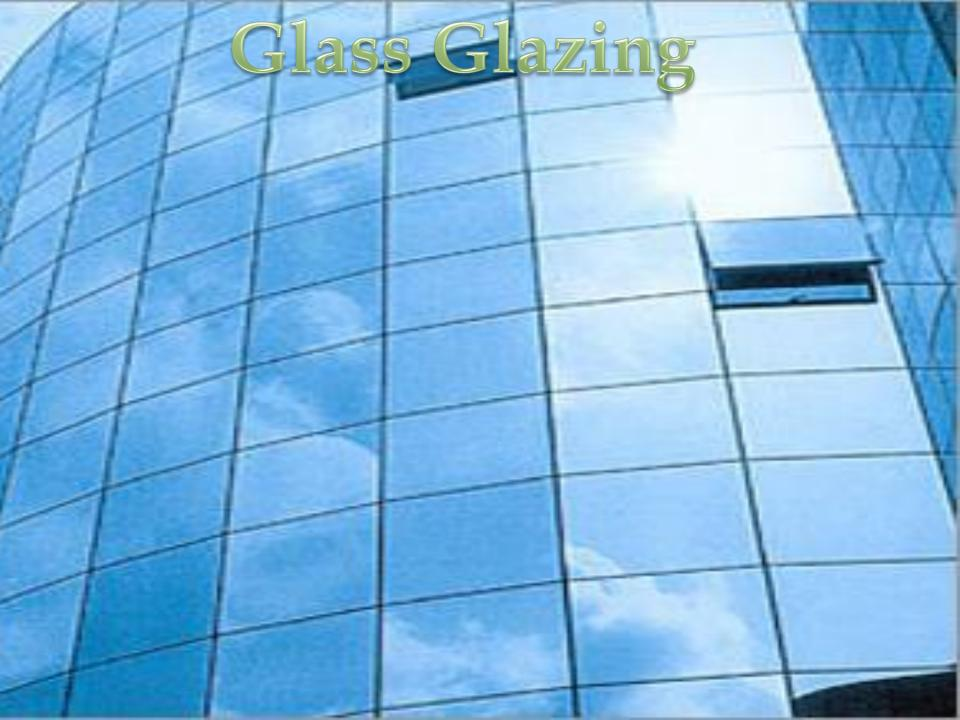
Distance between the external wall (glass / brick) and glass façade shall not be more than 300 mm. The smoke seals / barriers between building wall and façade shall be provided at every floor level in the form of non-combustible material / vermiculate cement.
